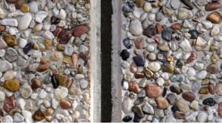
The expansion behavior of the tape depends on the joint and ambient temperature.
