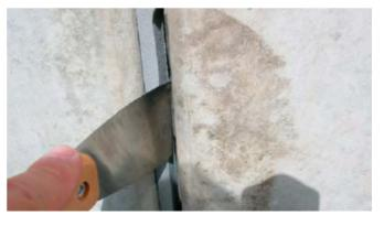
Due to security reasons the tape should be recessed in the joint by at least 2 mm from any radius or edge. The tape must not line up precisely with the edges of the joints!
